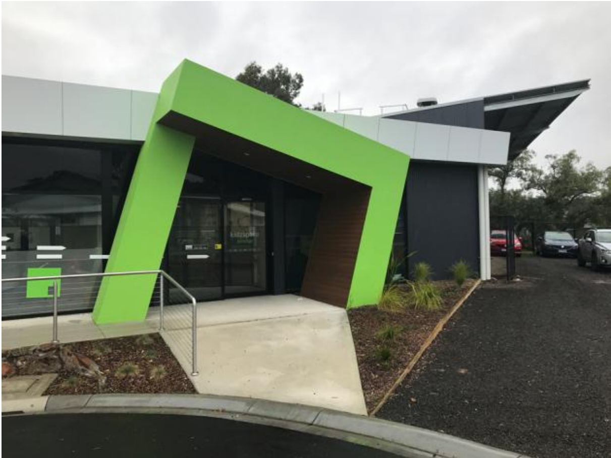
Figure 2 BCHS Kidzspace building
